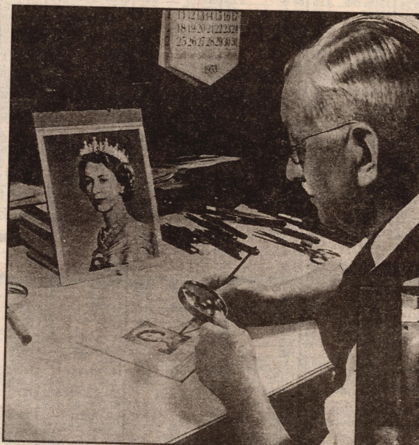
Figure 4: Siderographer transfers the stamp image to the printing plate.
